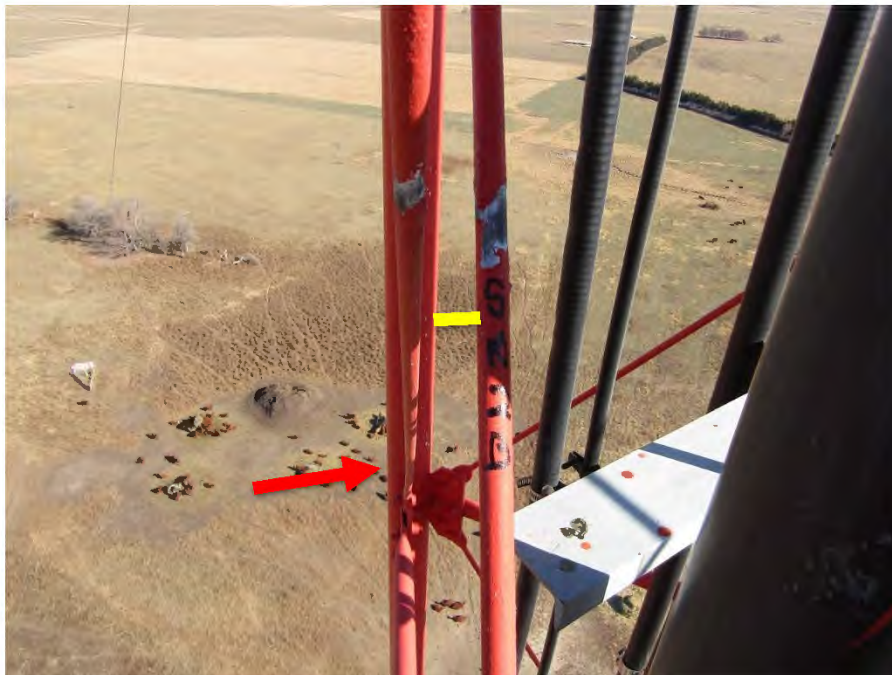
Bent diagonal member in Section #10 with 1" deflection. Photo also shows rust at the intersection of the diagonal members.
