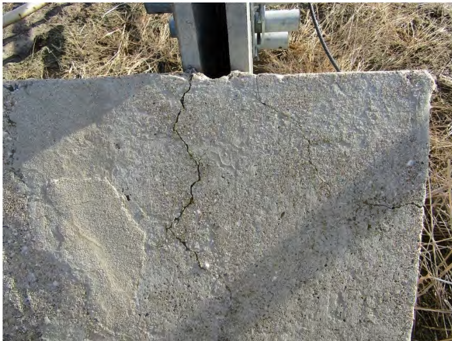
Small cracks in the concrete at the outer anchor C.
