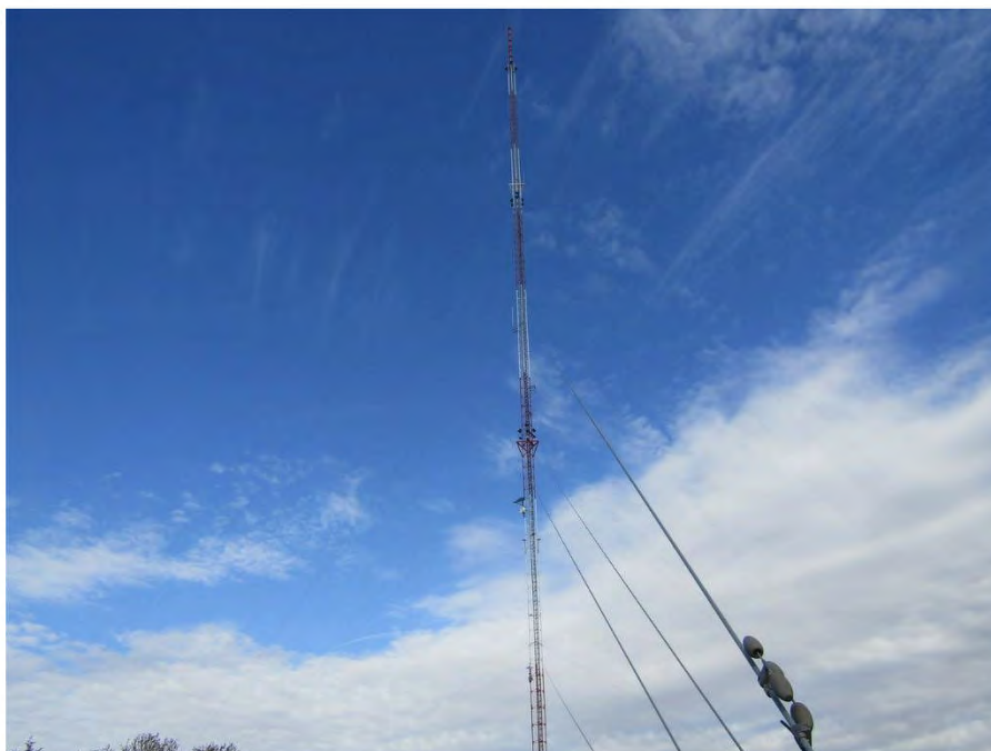
Profile view of tower.
