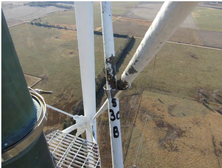
Typical loose banding at the intersection of diagonals. Photo also shows rust at the intersection of the diagonal members.
