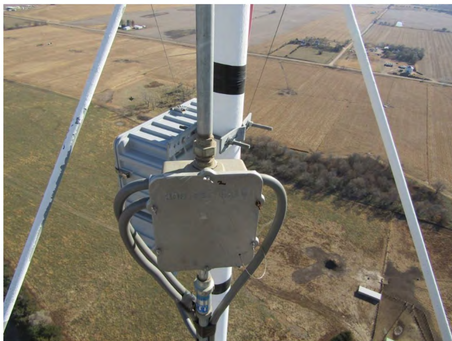
Junction box at light level #2.
