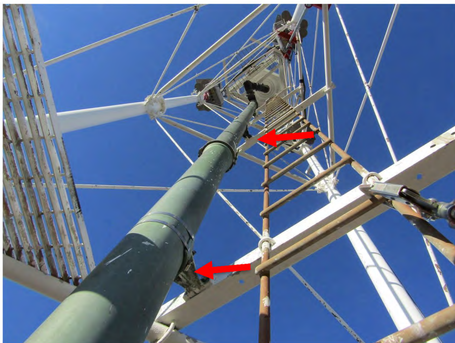
Fixed hangers below the top elbow complex. Photo also shows some surface rust on the ladder.
