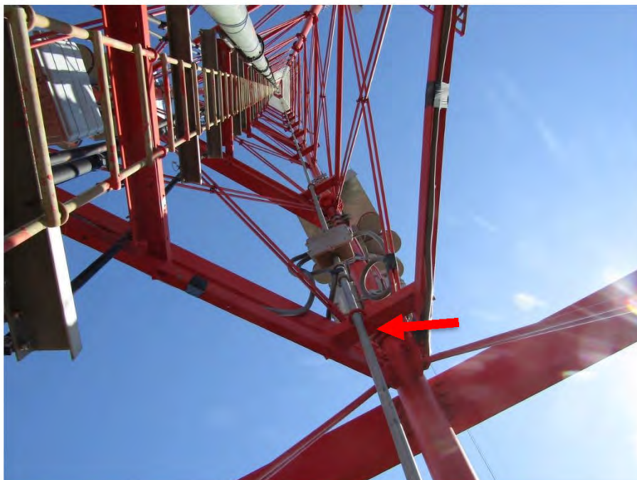
Location of rigid conduit in the tower.
