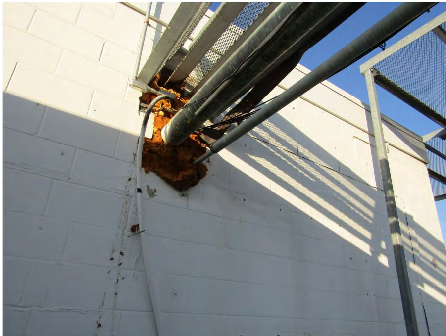
Transmission line entering the building.
