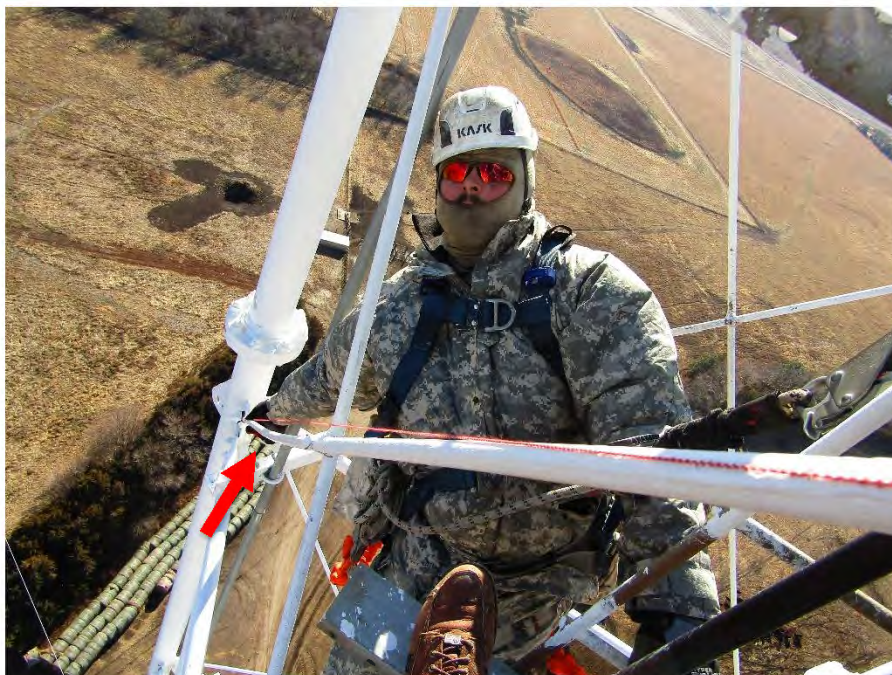
Bend at the lower end of diagonal member in Section #15.
