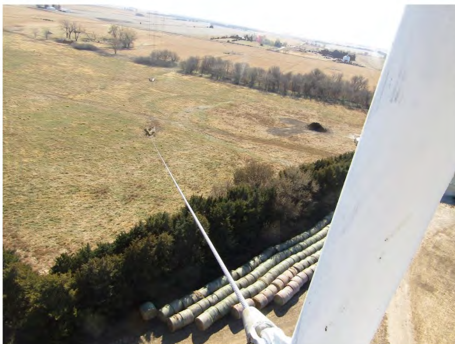
Typical tower connection for guy wires at levels #1, #3, #5, & #6.
