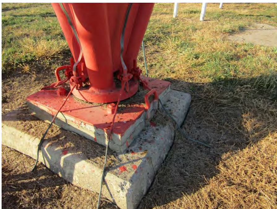
Grounding at the tower base.
