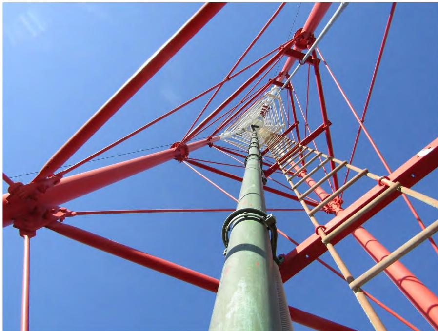
Transmission line location in the tower.
