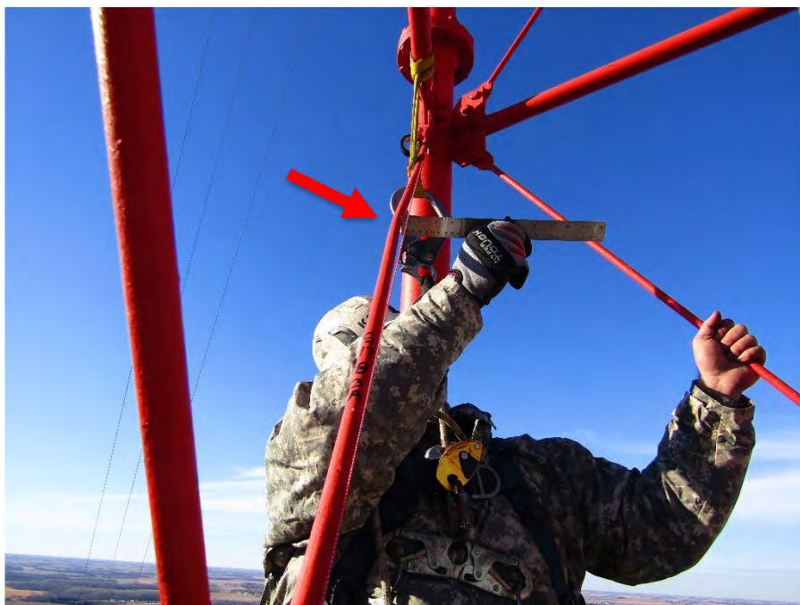
Bent diagonal member in Section #17.
