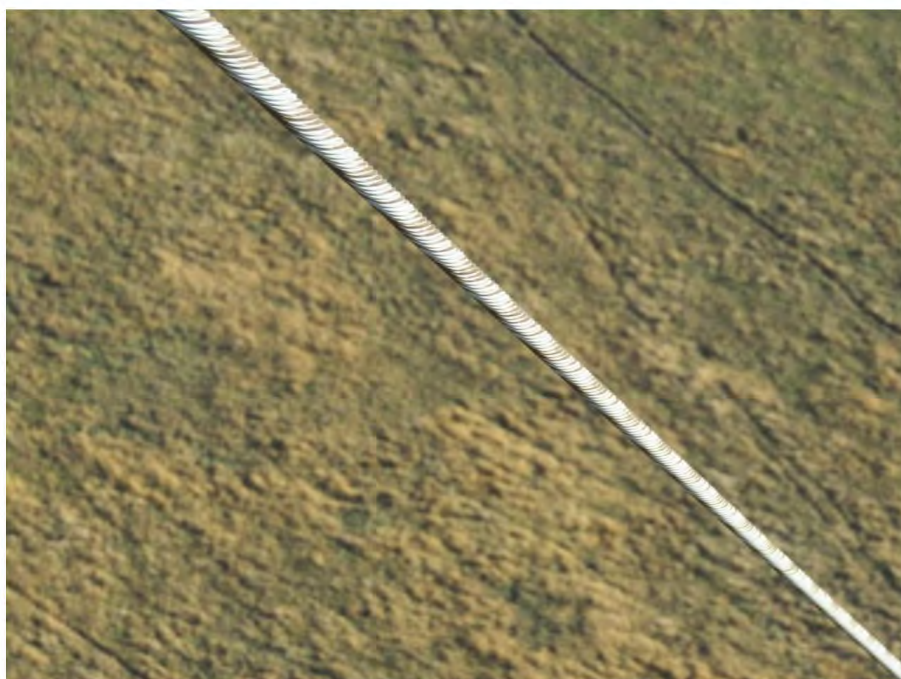
Typical areas of surface rust on a level #6 guy wire.
