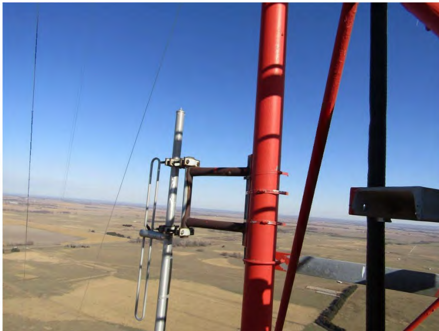
Surface rust on the mount for the dipole antenna in section #20.
