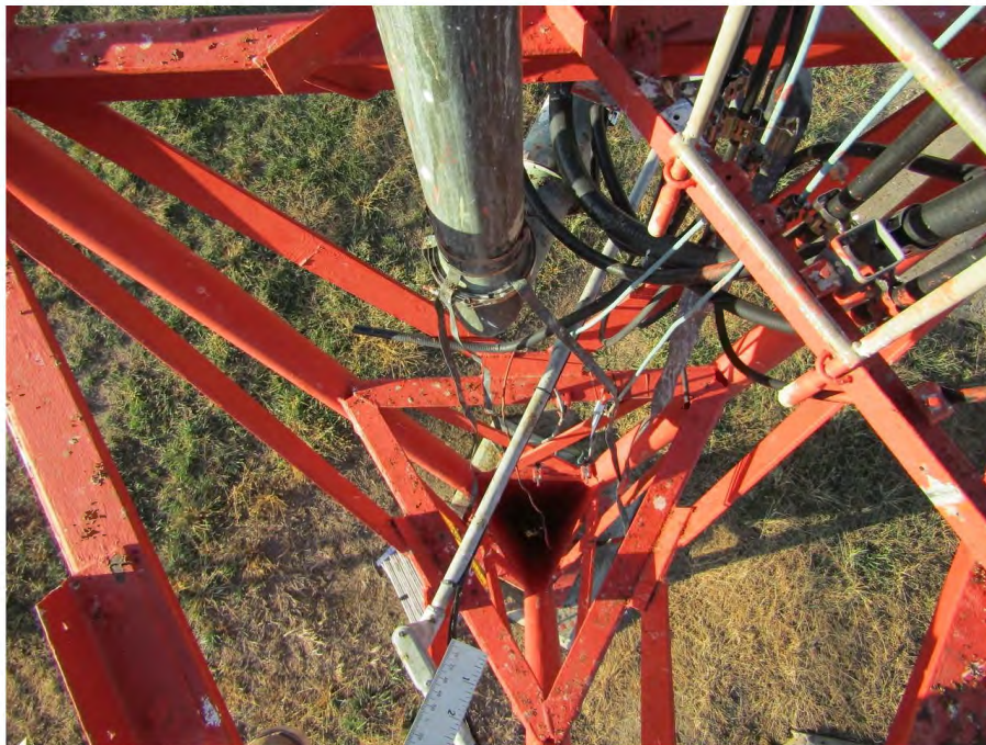
Transmission line elbow complex at the tower base.
