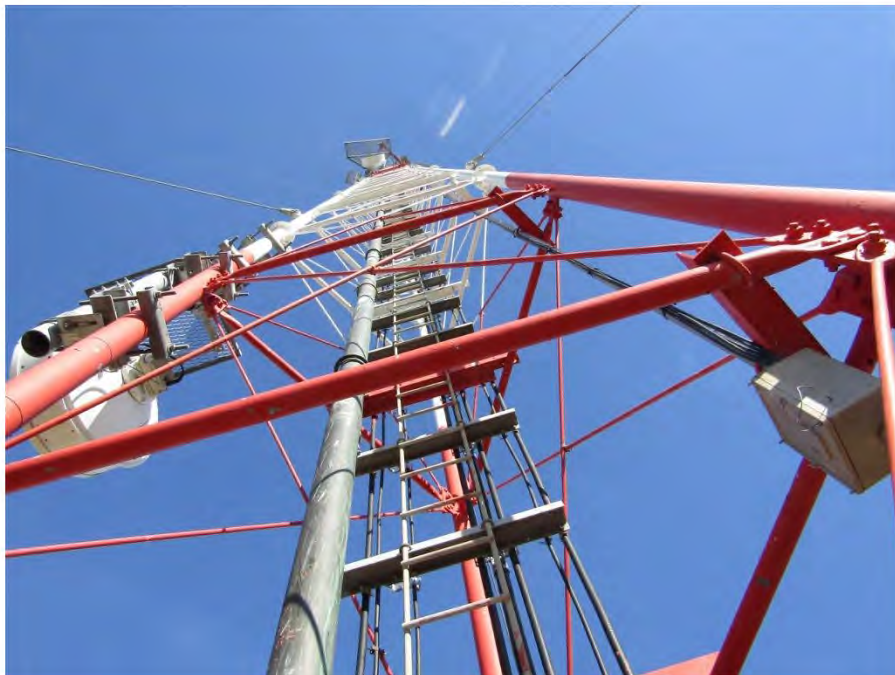
The climbing ladder without a safety climb cable system. Photo also shows C-channel brackets secured to the back side of the ladder.
