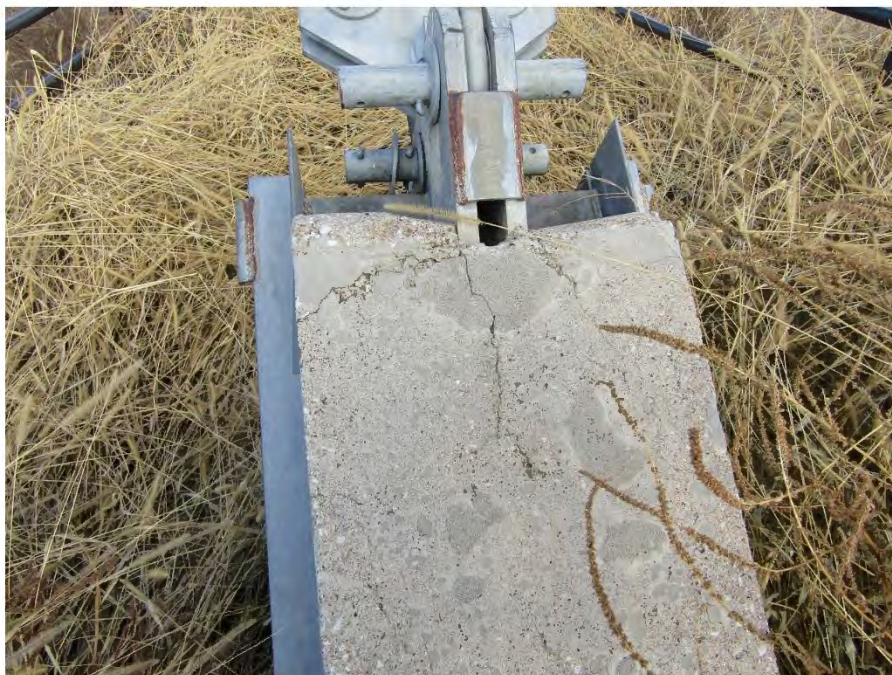
Small cracks in the concrete at the inner anchor B.
