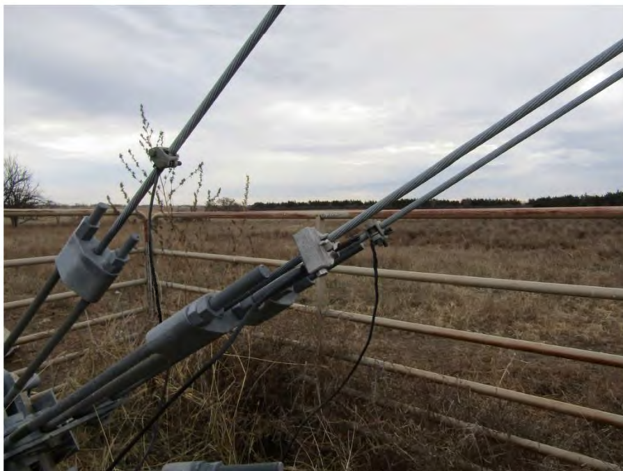
Typical grounding cable connections on guy wires.
