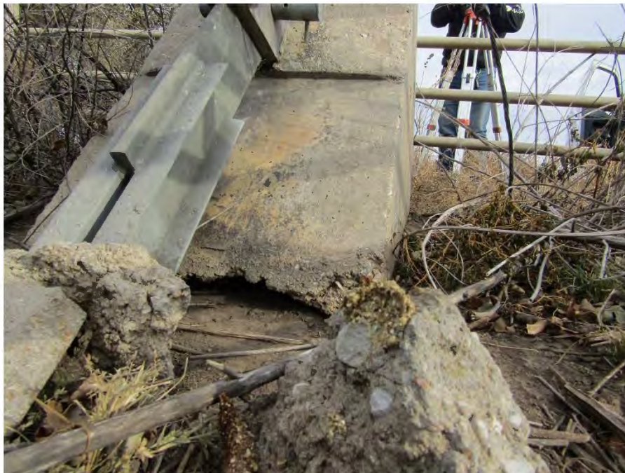
Broken concrete at the outer anchor A.
