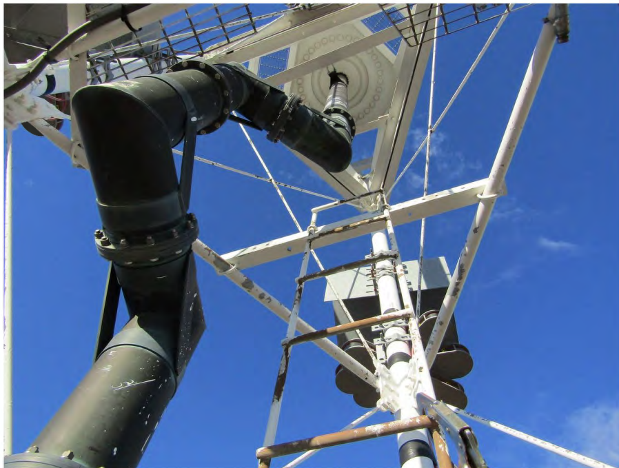
Transmission line elbow complex below the antenna input. Photo also shows some surface rust on the ladder.
