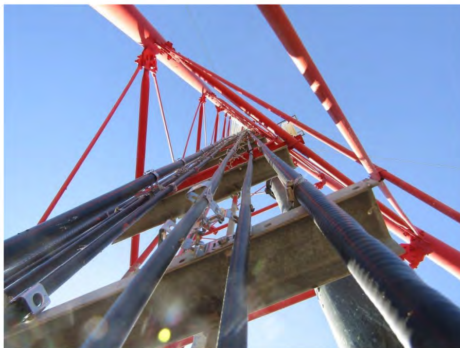
Flexible lines to ancillary systems
