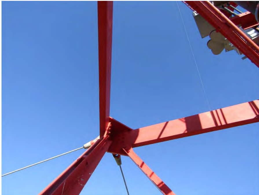
Typical tower connection for guy wires at double guyed levels #2 & #4.
