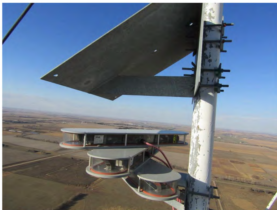
Typical flash head and ice shield.
